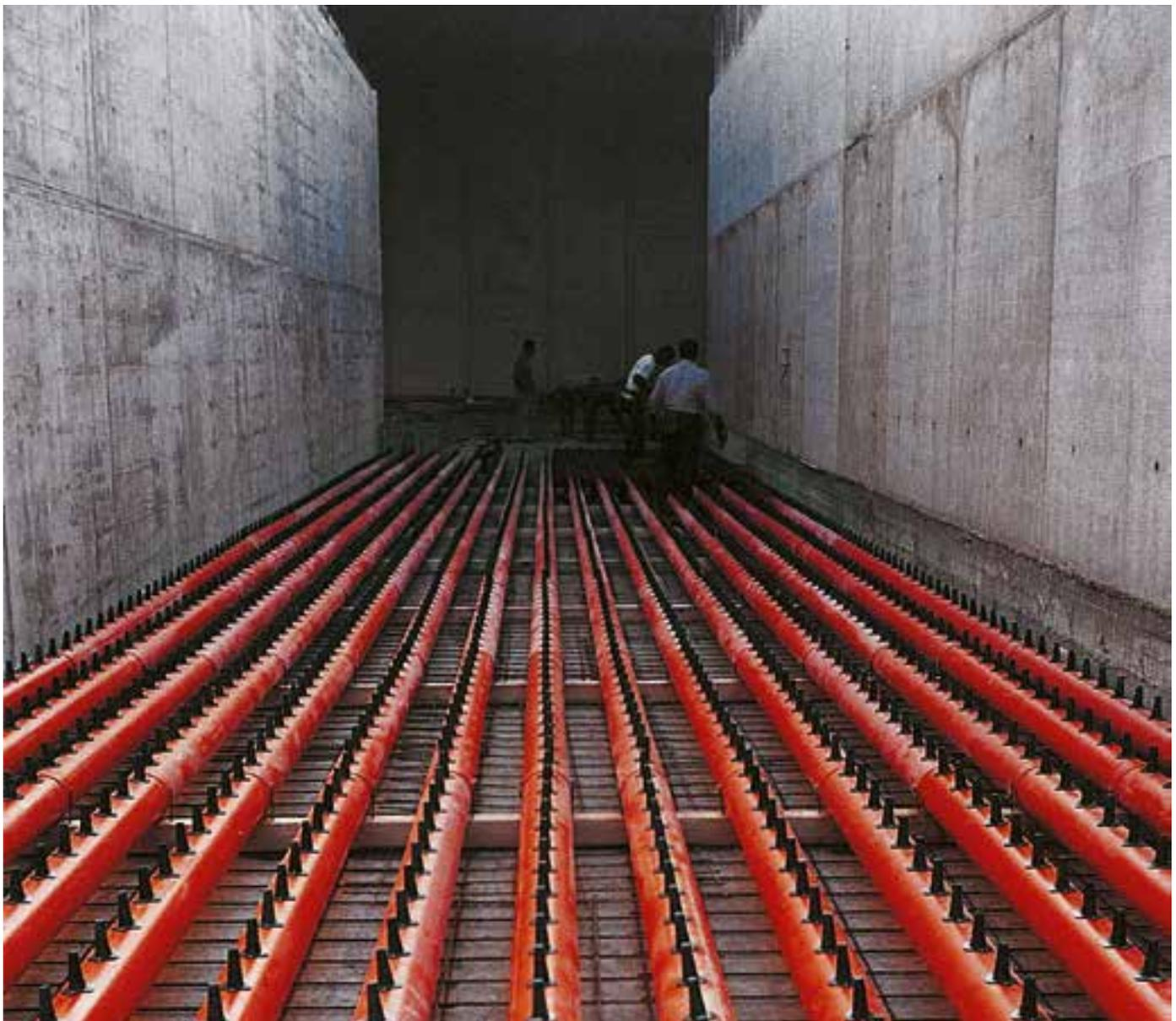
The plant uses tunnel composting technology developed by Ecomaster for treating organic waste biologically in order to hygienize and stabilize it. The process takes place in modular, closed reactors consisting of reinforced concrete tunnels equipped with a ventilation system integrated in the floor.
