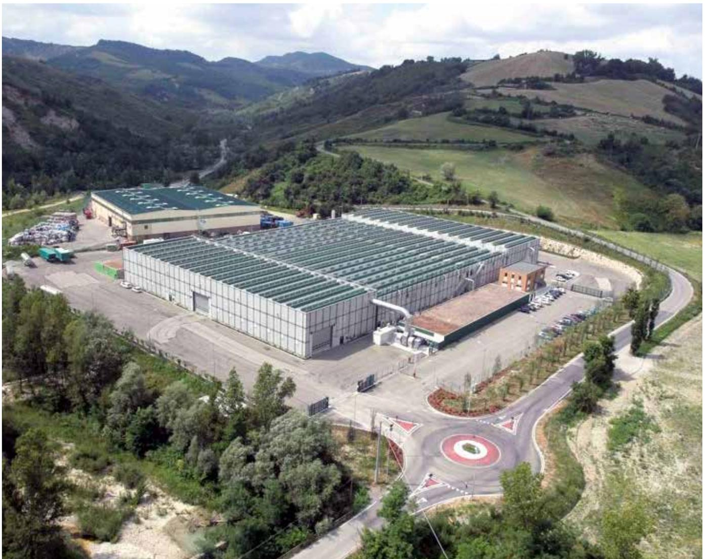
The plant uses a combination of anaerobic (digestion) and aerobic (composting) processes for the treatment of organic waste with recovery of electric energy and compost.
