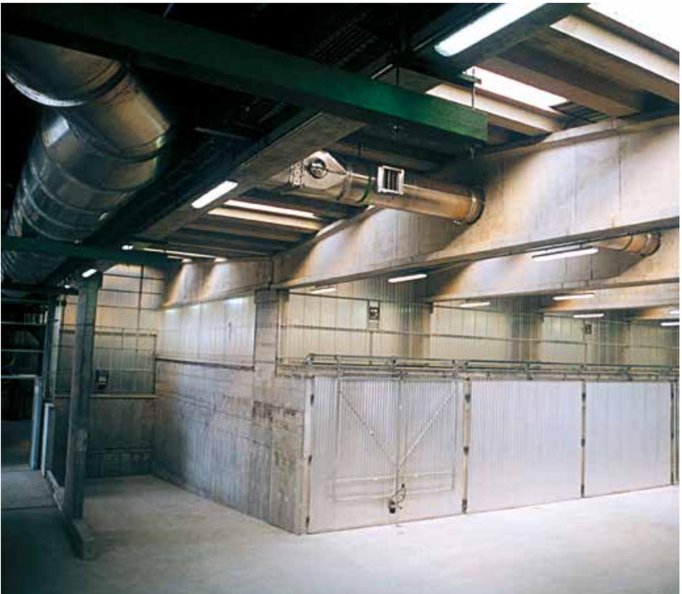
The plant uses tunnel composting technology for biological treatment of source-separated organic waste in order to hygienize and stabilize it, which, after the curing phase, produces quality compost. The process takes place in five closed reactors, consisting of reinforced concrete tunnels equipped with a ventilation system integrated in the floor.
