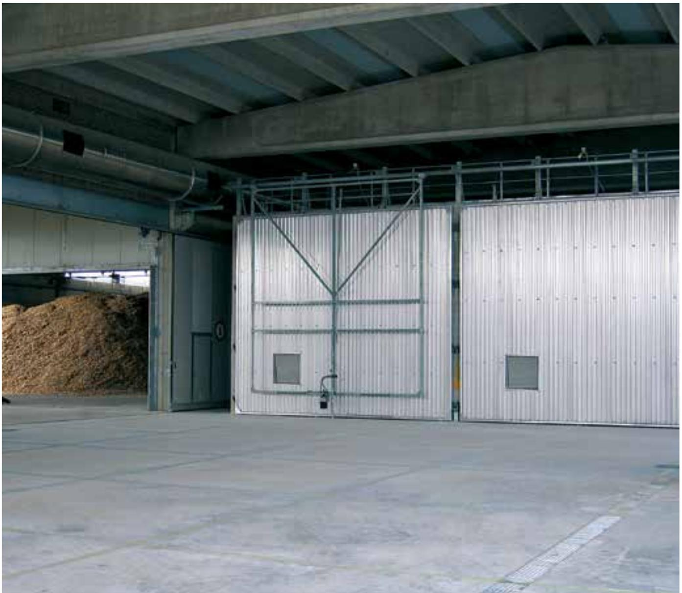
The plant uses tunnel composting technology for biological treatment of source-separated organic waste in order to hygienize and stabilize it, which, after the curing phase, produces quality compost. The process takes place in three closed reactors, consisting of reinforced concrete tunnels equipped with a ventilation system integrated in the floor.
