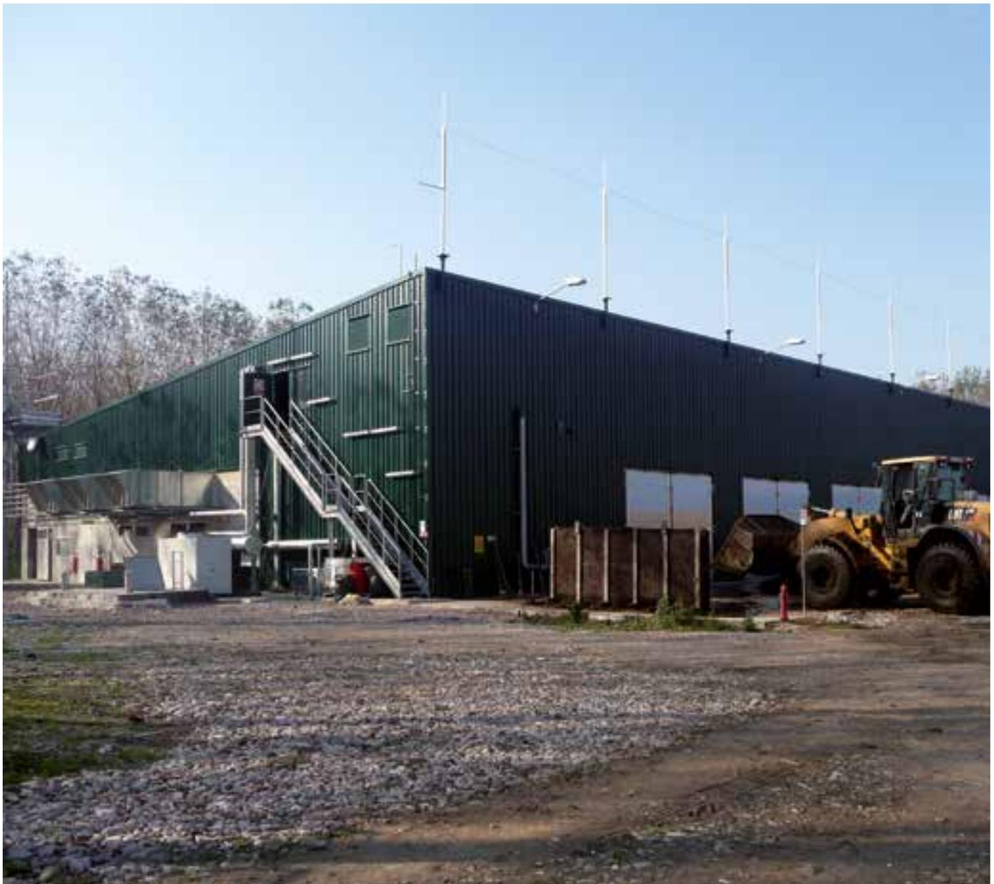
The treatment plant of bovine manure and corn silage, created in San Canzian d'Isonzo, uses the process of dry anaerobic digestion, developed in a battery of fermenters arranged in a parallel formation.
