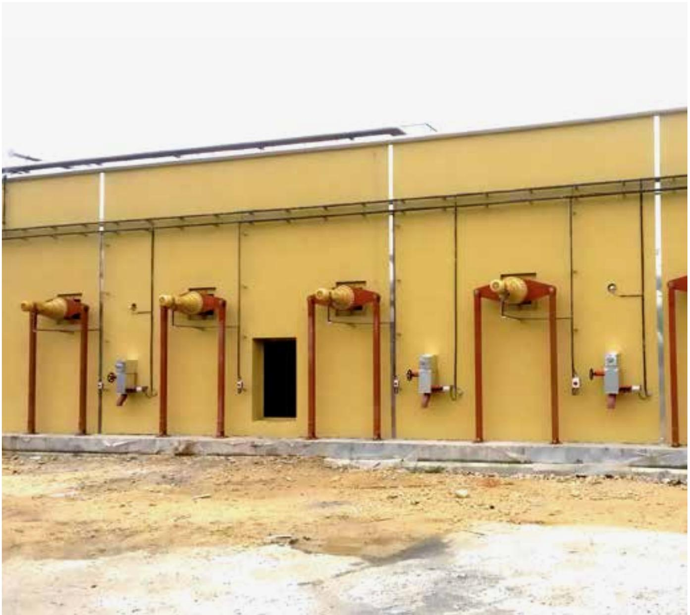
The digester used for this application is substantially a construction made of reinforced concrete having a parallelepiped shape. The walls and the roof of the digester are insulated and a heating system is provided internally for maintaining the required process temperature.
