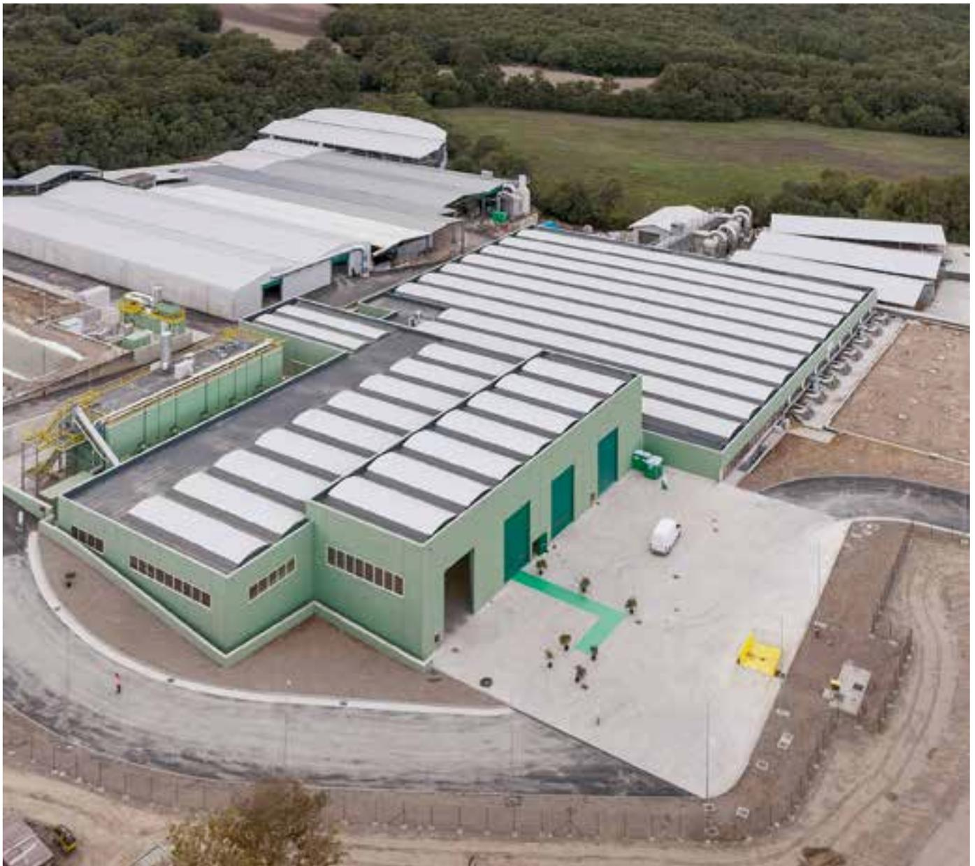
Source separated organic waste is processed by a pre-treatment line for sorting the organic components to be digested from rejects consisting of plastic bags and other non-biodegradable waste. The organic material produced in the pre-treatment line is then mixed with shredded green waste, which acts also as a bulking agent for the digestion process. The bulking agent derives from green waste shredding and compost screening operations.
