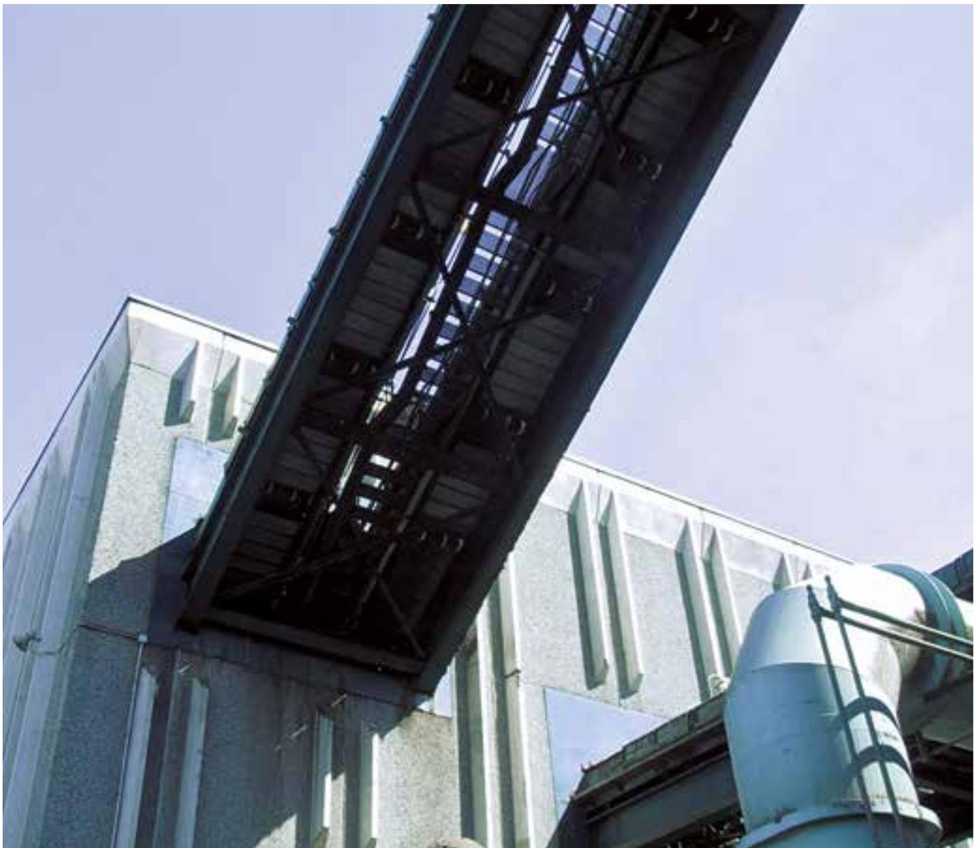
The feeding line of the second boiler consists of various long belt conveyors that connect the RDF receiving building with the storage area located nearby the boiler. The flexibility of the design is such that RDF can be received and stored in both areas depending on the operational requirements.
