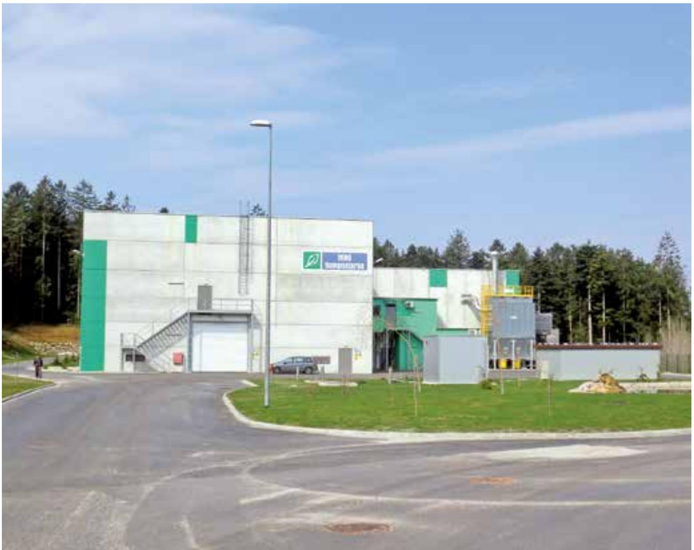
The project involves the construction of a facility with a section for aerobic stabilization of organic source separated waste and another section for stabilization and mechanical treatment for mixed municipal waste aimed at the recovery of material.
