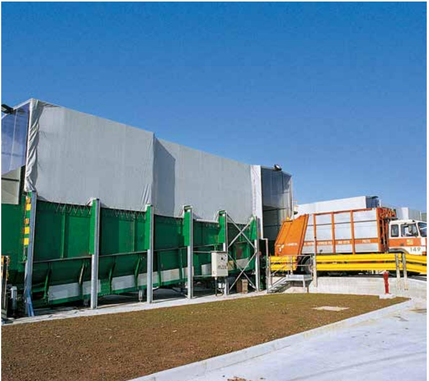
In Padua municipal solid waste collected by compactor trucks is taken to a transfer station, where waste is loaded into trailer trucks that transport it to a sanitary landfill.
