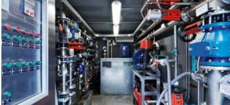
Type of project: New containerized WWTP (42 mc/h) Electromeccanical and hydraulic installation of a prefabbricated MBR system.
